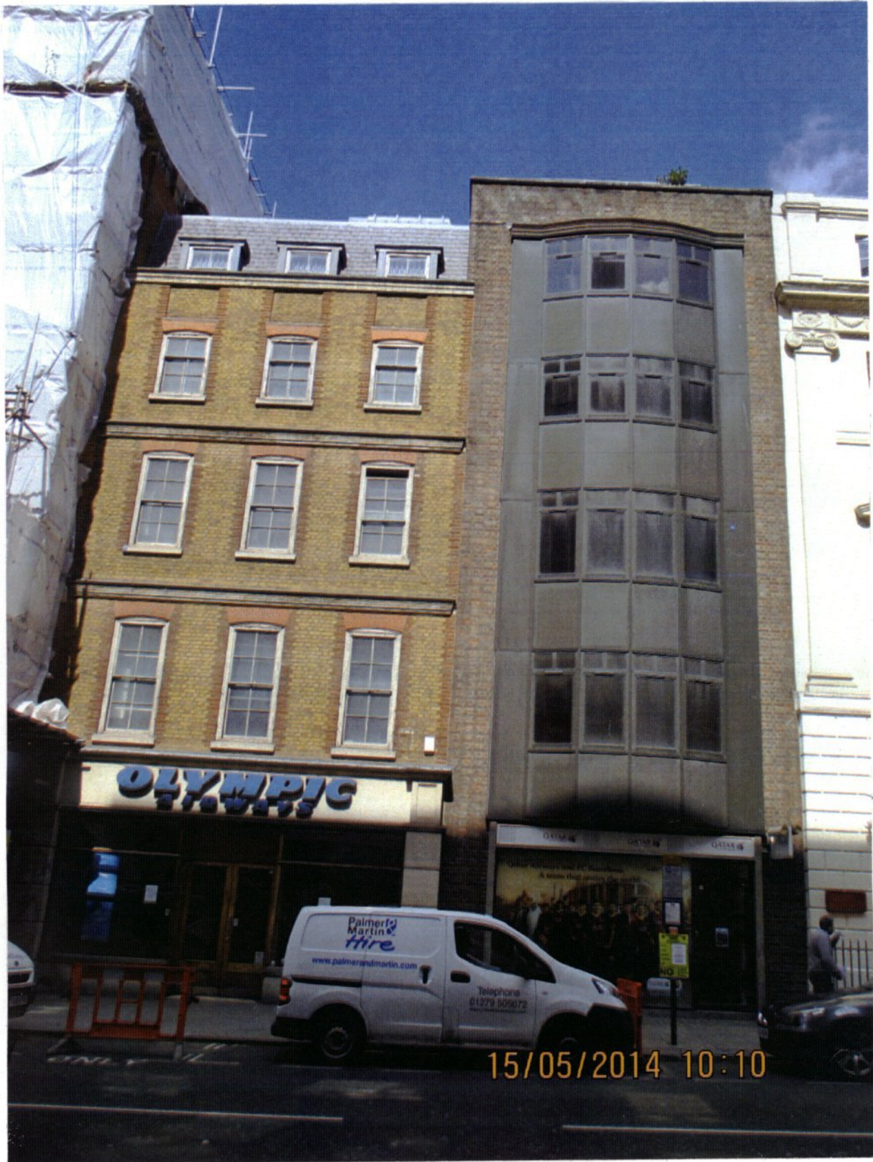
10 and 11 Conduit Street, W1
